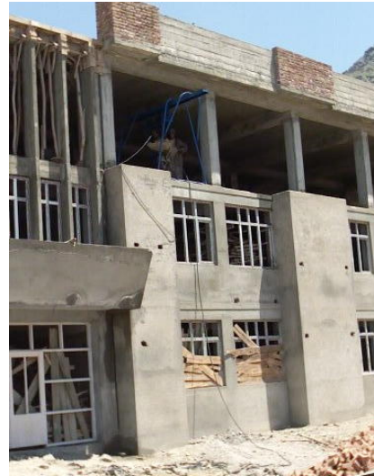
Two years' construction results at the Omara Khan School in Kabul
